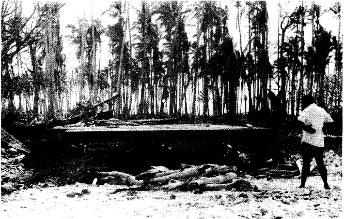
A complete house was blown off its platform during Cyclone Namu because of a lack of structural continuity between the walls and the floor.
