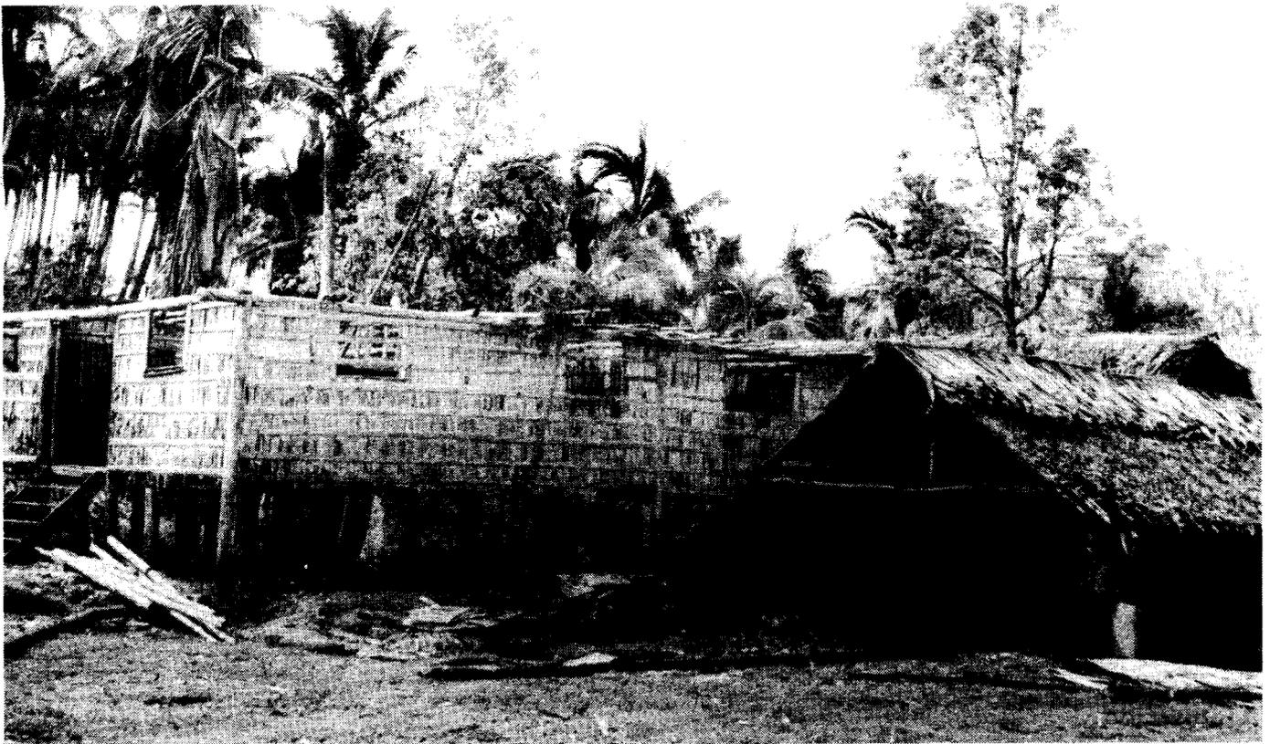
TRADITIONAL HOUSING IN THE SOUTH PACIFIC - A new house loses its roof during a cyclone while an older house remains standing.
